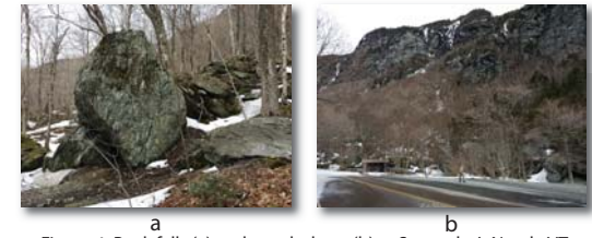
Figure 4. Rock falls (a) and a rock chute (b) at Smuggler's Notch, VT.
